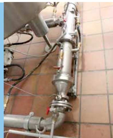
The KNOLL MX30S progressing cavity pump has been fitted with a double-walled, welded jacket at the request of Ritter Sport.
