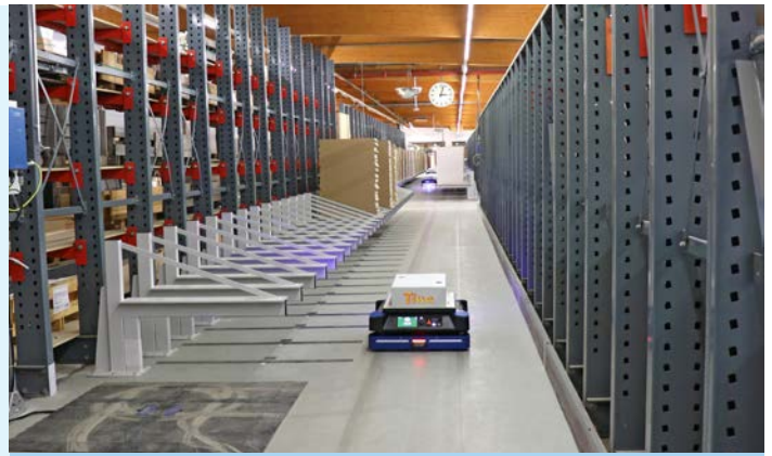
Buffer stations arranged in a row. A total of 137 places are now available.
