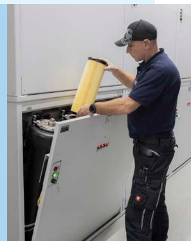
Maintenance Manager Horst Anger demonstrates how easy it is to replace the filter cartridges.
