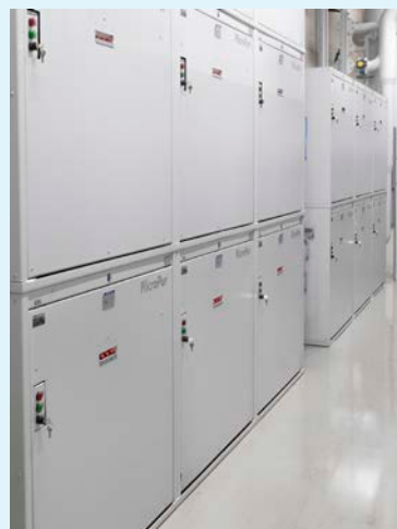
Fifteen modules of the standard MicroPur® 480 M filter were installed in the first expansion stage. Each module contains four housings, each equipped with two cartridges. These can be changed in just one or two minutes – easily and without dripping.
