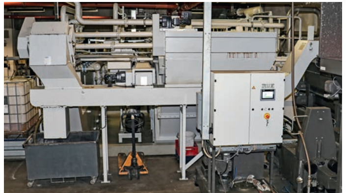
After cleaning, the grinding sludge discharged is pressed into pellets and the recovered cooling lubricant is fed back into the circuit.
