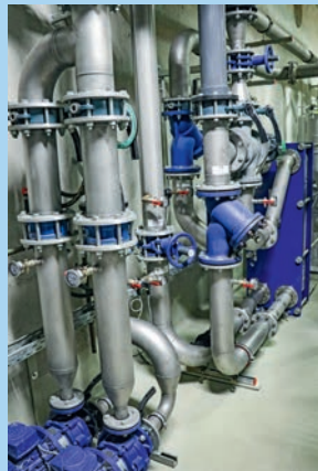
Pipework of the cooler/plate heat exchanger.
