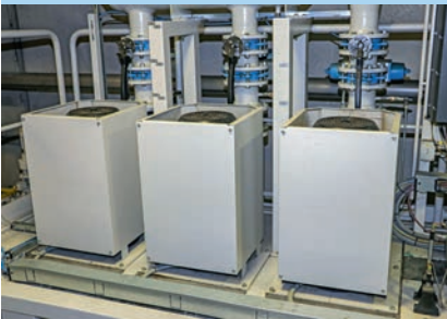
Frequency-controlled clean coolant pumps with noise protection hoods.
