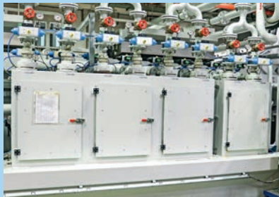
The essential filter capacity is provided by four hydrocyclones (in housings due to the aerosol formation). Under these is the collecting conveyor for the sludge from the cyclones and over these, the piping for the cyclones.
